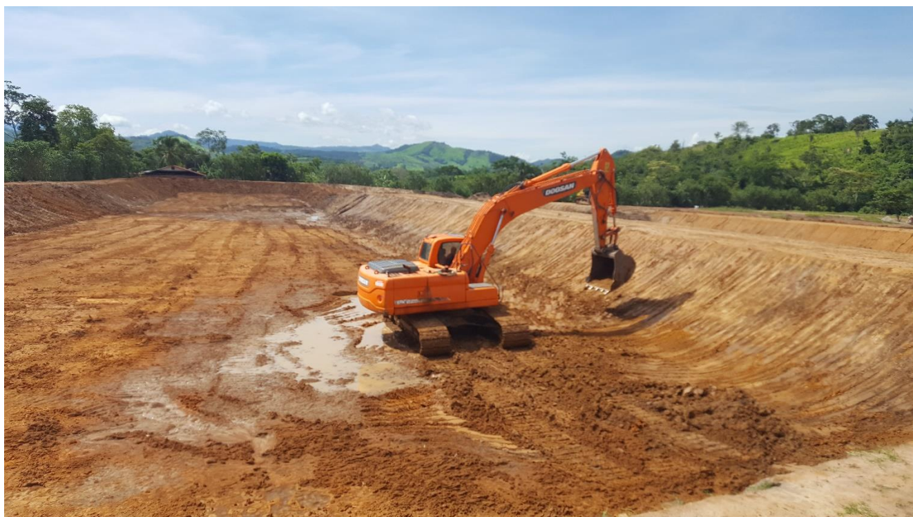
Picture 4: Construction 2 reservoir ponds which will supply water to the Tilapia nursing ponds with green water
